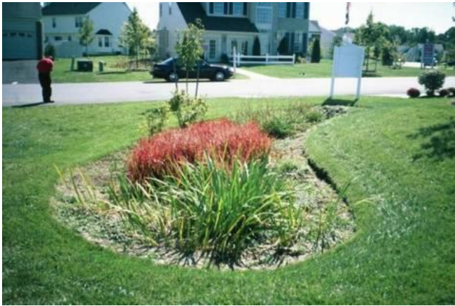
Figure 5.1.a – Bioretention System
