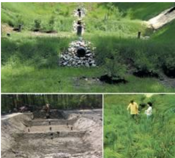
Figure 5.2.b – Subsurface Gravel Wetlands (UNHSC)
