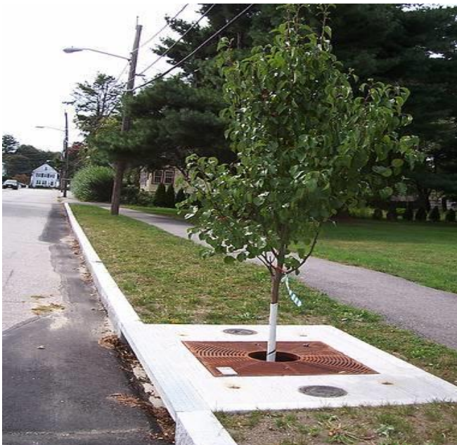
Figure 5.1.b – Filterterra Tree Filter ( www.filterterra.com )
