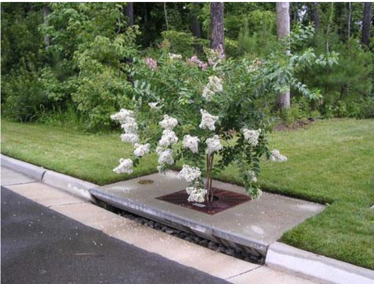
Figure 3.5.d – Filterra Bioretention (Filterra.com)
