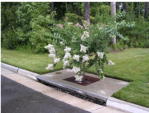
Figure 5.5.d – Filterra Bioretention (Filterra.com)
