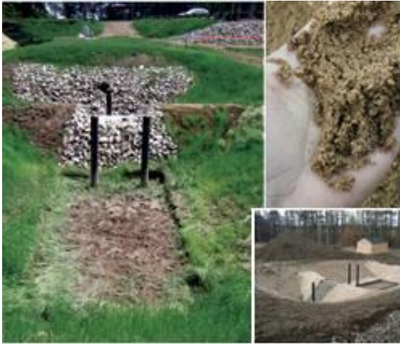
Figure 5.1.c – Surface Sand Filter (UNHSC)
