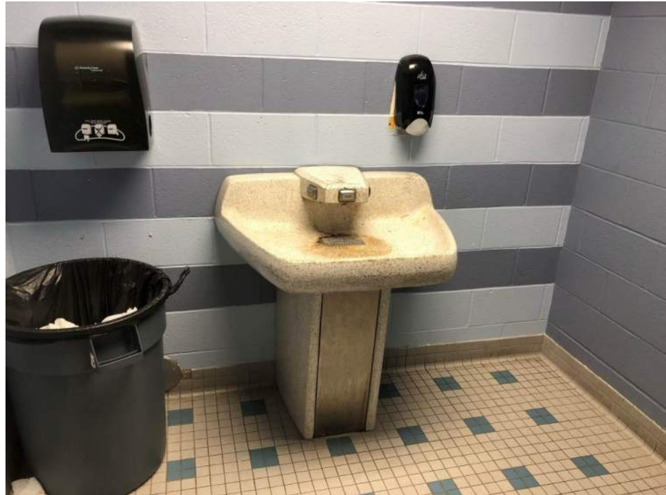
Existing Bradley lavatory in one of the boys bathrooms.
