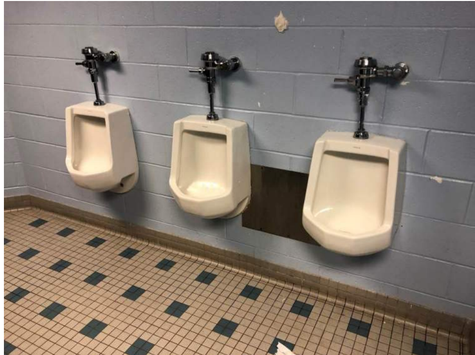
Existing urinals in one of the boys bathrooms.
